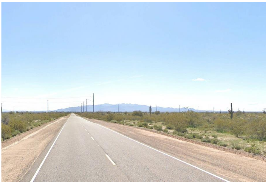
View 19 , looking south from 211 th Avenue
