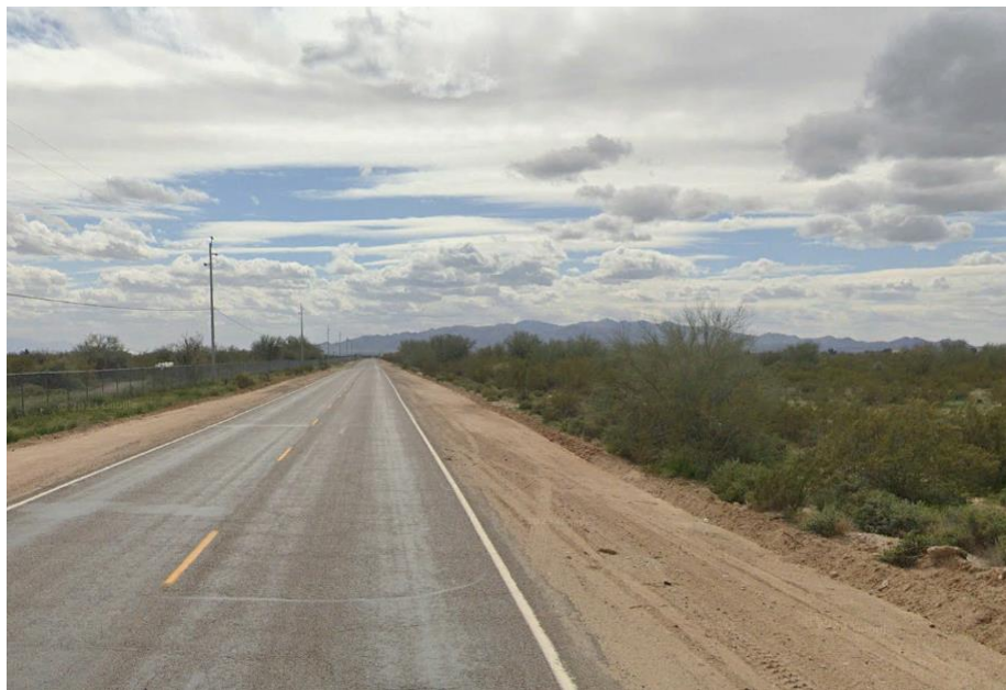
View 11 , looking south from 211 th Avenue
