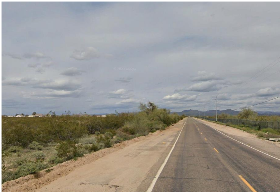
View 9 , looking north from 211 th Avenue
