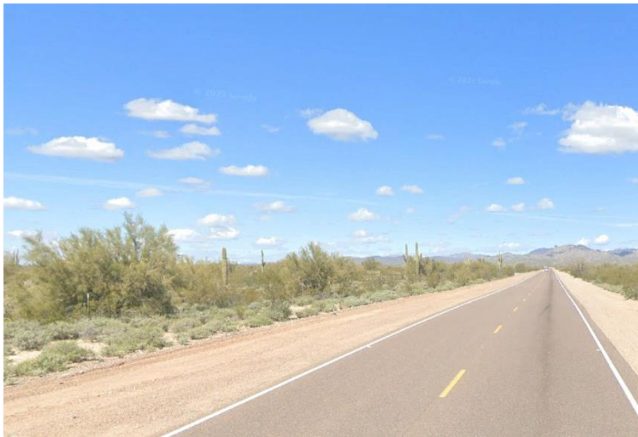
View 17 , looking north from 211 th Avenue
