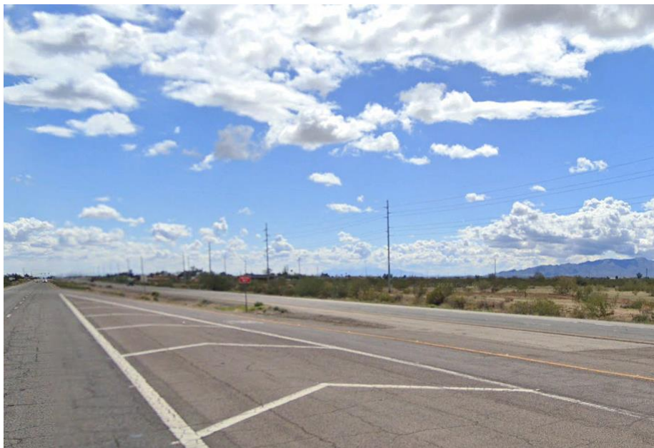
View 7 , looking southeast from US-60
